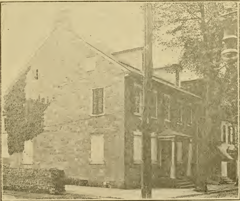
JOHN NICHOLAS' HOTEL ERECTED 1806 SECOND AND FERRY STREETS (Photo 1911)
