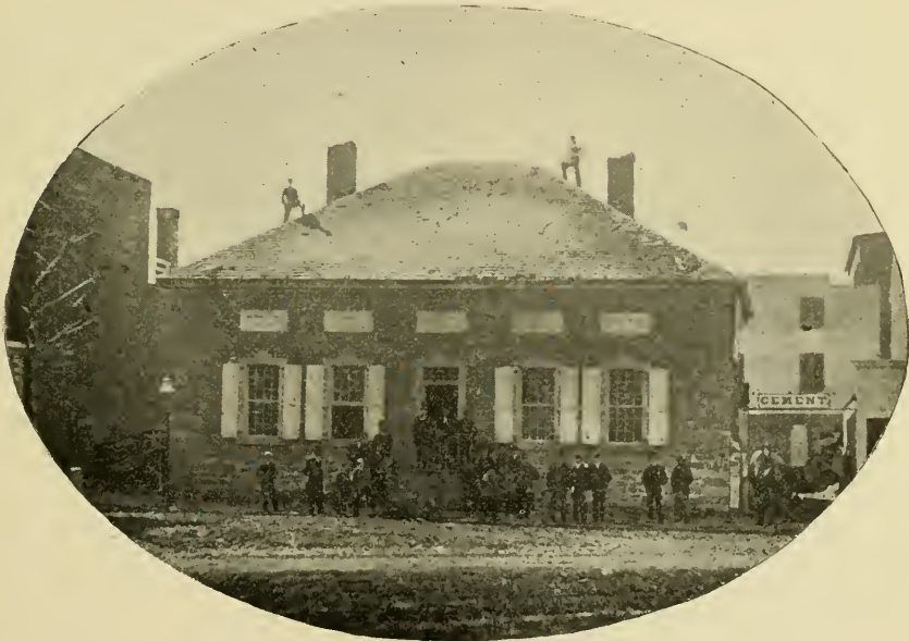
Old County House Demolished 1868.
