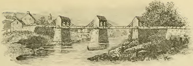
CHAIN BRIDGE OVER THE LEHIGH RIVER
