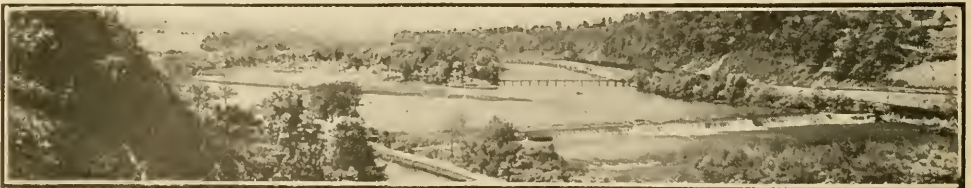
VIEW UP THE LEHIGH SHOWING CHAIN DAM AND ISLAND PARK
